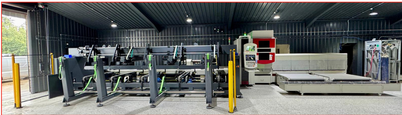
FULL MACHINE INSTALLATION
