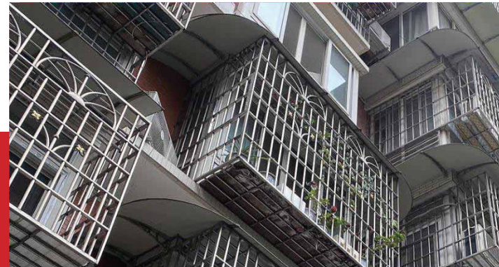
Metal Guardrails, Doors, and Windows
